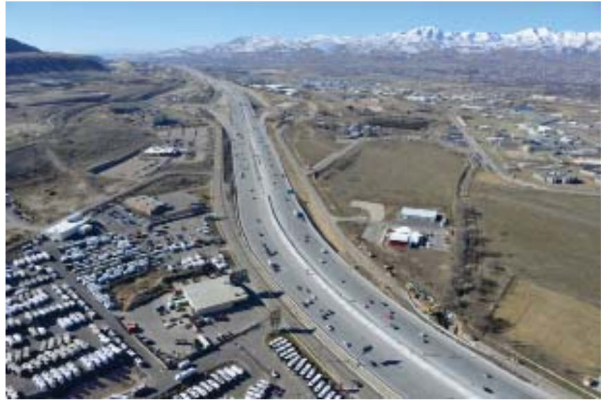
I-15, The Point Design-Build Project, Salt Lake City, UT
