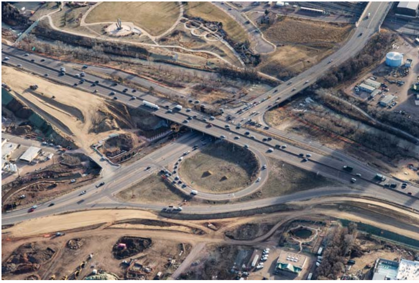
I-25/Cimarron Design-Build Project Colorado Springs, CO
